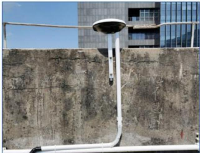
④ Installed antenna feeder joints, GPS antenna feeder joints, and other independent exposed cable joints, should be strictly in accordance with the "1 + 3 + 3" treatment (1 layer of insulation tape + 3 layers of waterproof tape + 3 layers of insulation tape wrapping) waterproof.
